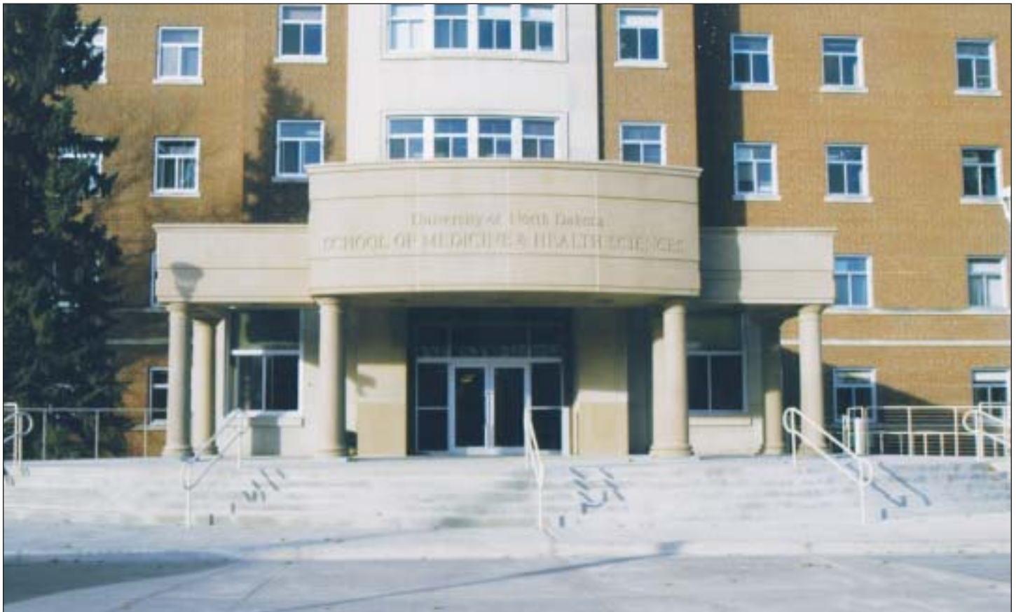
The new facade of the UND School of Medicine and Health Sciences features an expansive concrete staircase flanked by permanent flower boxes. Columns grace the approach which also includes a ramp for handicap-access and heavy glass doors.
